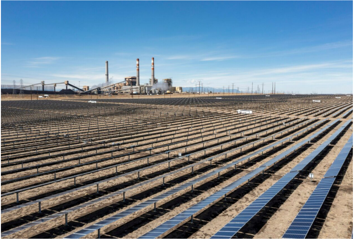
Evraz Rocky Mountain Steel, the largest electricity consumer in Colorado, is now getting much of its power from an immense solar farm next door. The farm was developed by Lightsource BP, half-owned by BP, the oil company.
