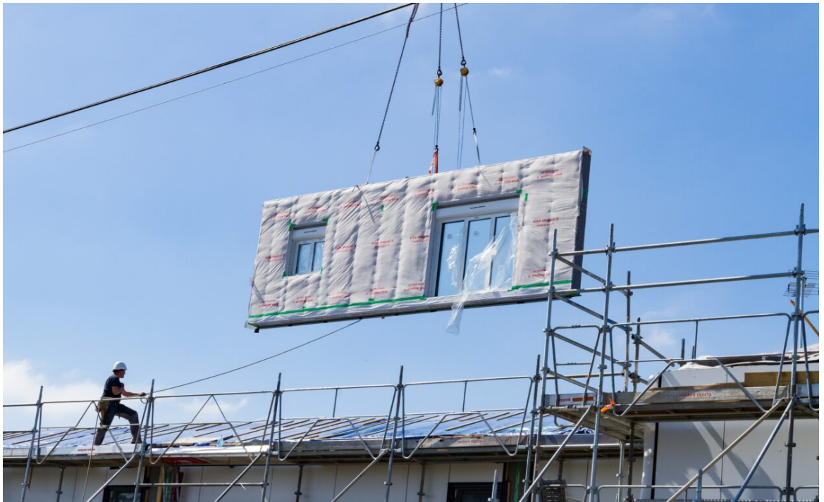
A worker manoeuvres into place a panel containing thermal insulation and advanced windows and doors, as old buildings in France are renovated to be more energy-efficient.
