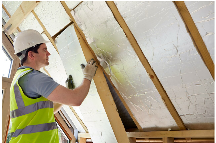
A new home gets high-quality insulation to save energy.
